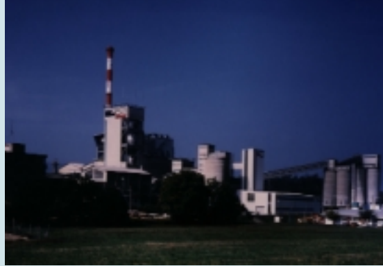
Photo of the HCB Cement Plant in Siggenthal
